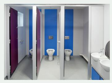
and changing cubicles in Solid Grade Laminate (SGL) as it's designed to meet the most stringent specifications of durability and hygiene.
