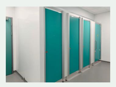
In addition to patient safety and durability, Venesta tailored the door widths to improve accessibility for all users. The washrooms were specified in our "Peacock" laminate to make their washrooms pop with colour. They featured a unique, adjustable pedestal which allows hassle-free cleaning from the outside of the cubicles.
