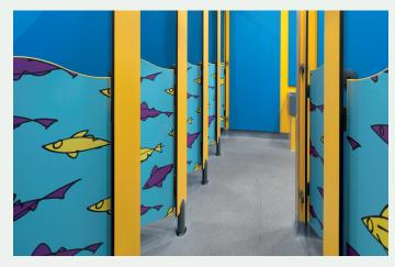
With an emphasis on balancing robust hygiene standards with cost-saving, the toilet cubicles were specified in the smooth and totally waterproof Solid Grade Laminate (SGL). Time and money were saved on the WC and vanity units by utilising Vepps, our pioneering IPS system. The sanitaryware was pre-plumbed onto High Pressure Laminate (HPL) panels, tested in our factory and delivered, ready for accurate and speedy installation.
