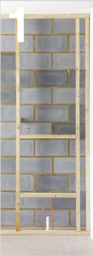
01 Install timber-frame (supplied by others).
