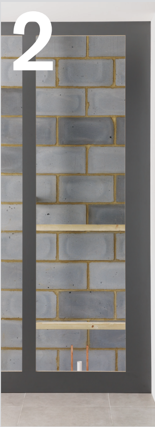
01 Install timber-frame (supplied by others).
